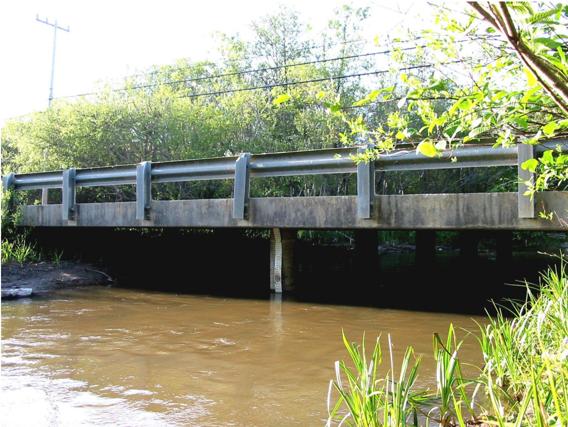
Pescadero Road Bridge after Beaver Dam Removal (Winter 2002)
