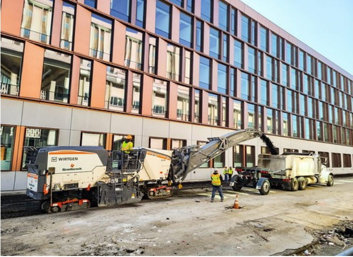
Construction of County Office Building 3 @ County of San Mateo
