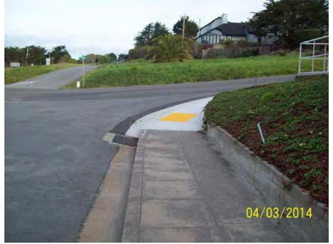
**Figure 2.** Existing storm drain catch basin at intersection of Carlos Street and Etheldore Street (looking north).
