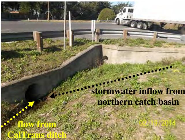
**Figure 5.** Pipe inlet for storm drain system outflow beneath Highway 1.
