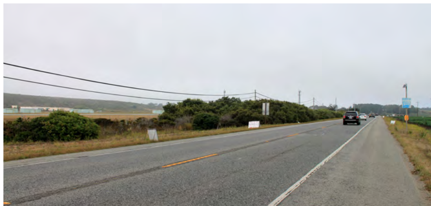
Existing overhead utilities along Highway 1
