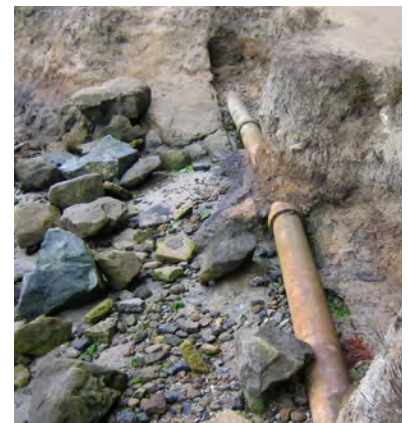
Erosion at the Terminus of Columbia Avenue (top) and Shoreline Erosion along the West Shoreline Trail (bottom)
