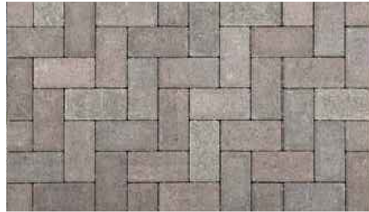
PERMEABLE PAVERS AT DRIVEWAYS (HERRINGBONE PATTERN)
