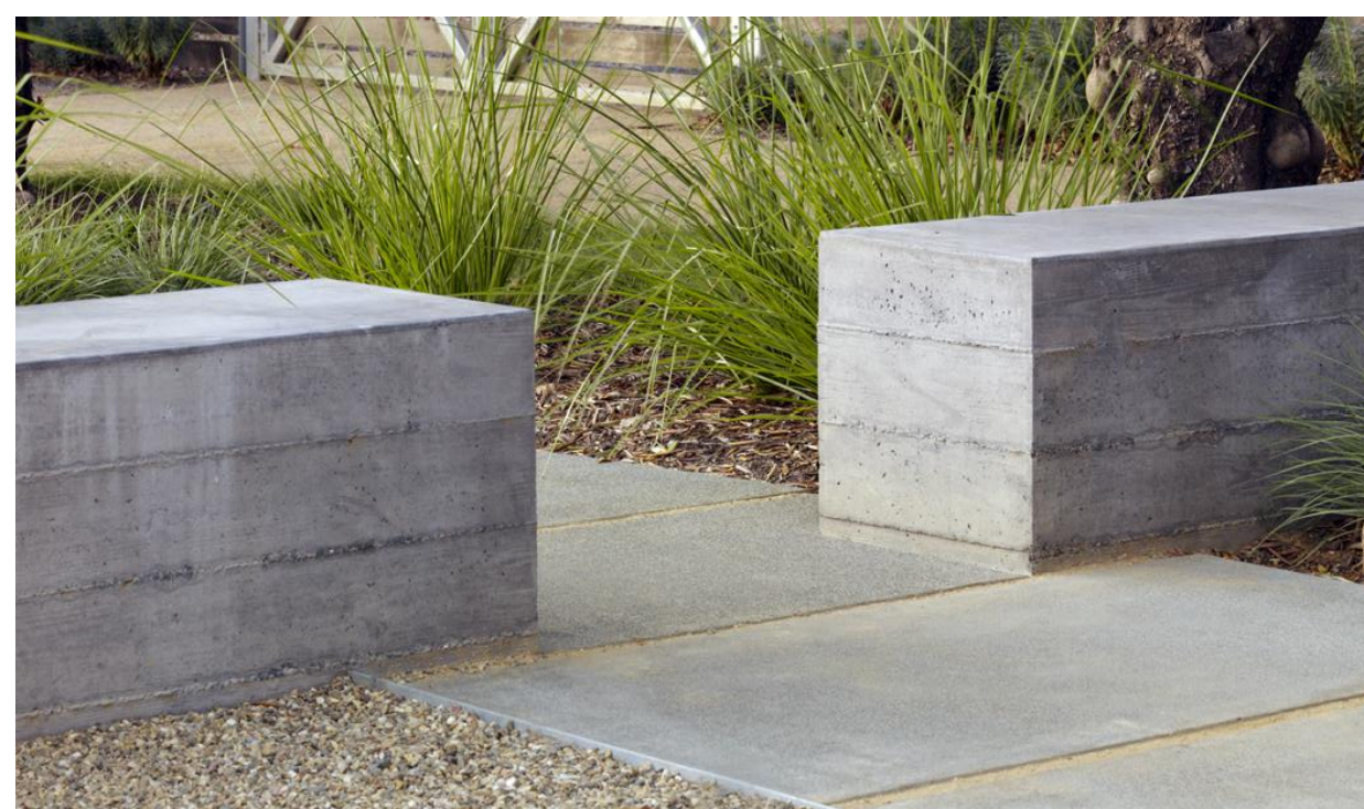
LANDSCAPE WALL AT DRIVEWAY (HORIZONTAL BOARD FORM FINISH)
