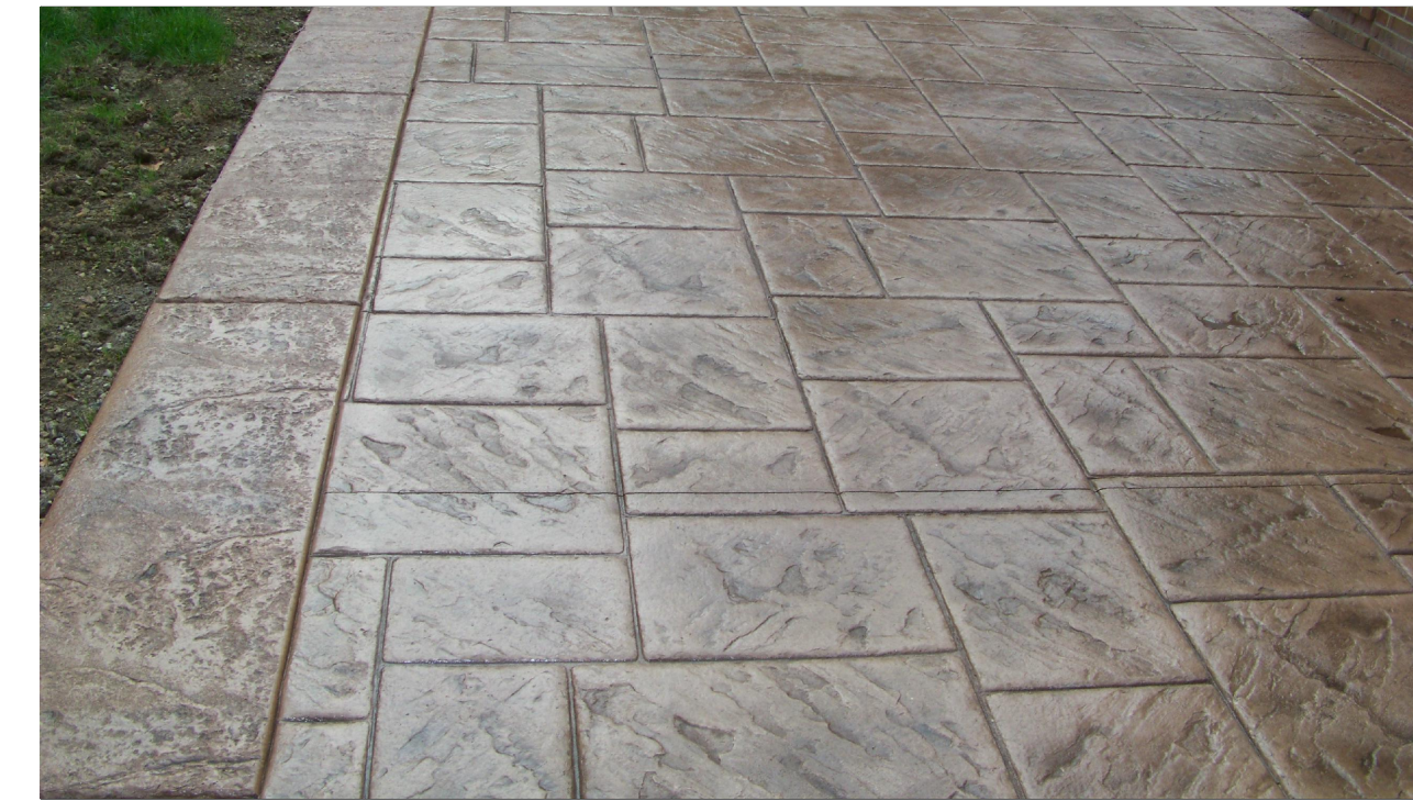
STAMPED CONCRETE AT DRIVEWAY ENTRANCES
