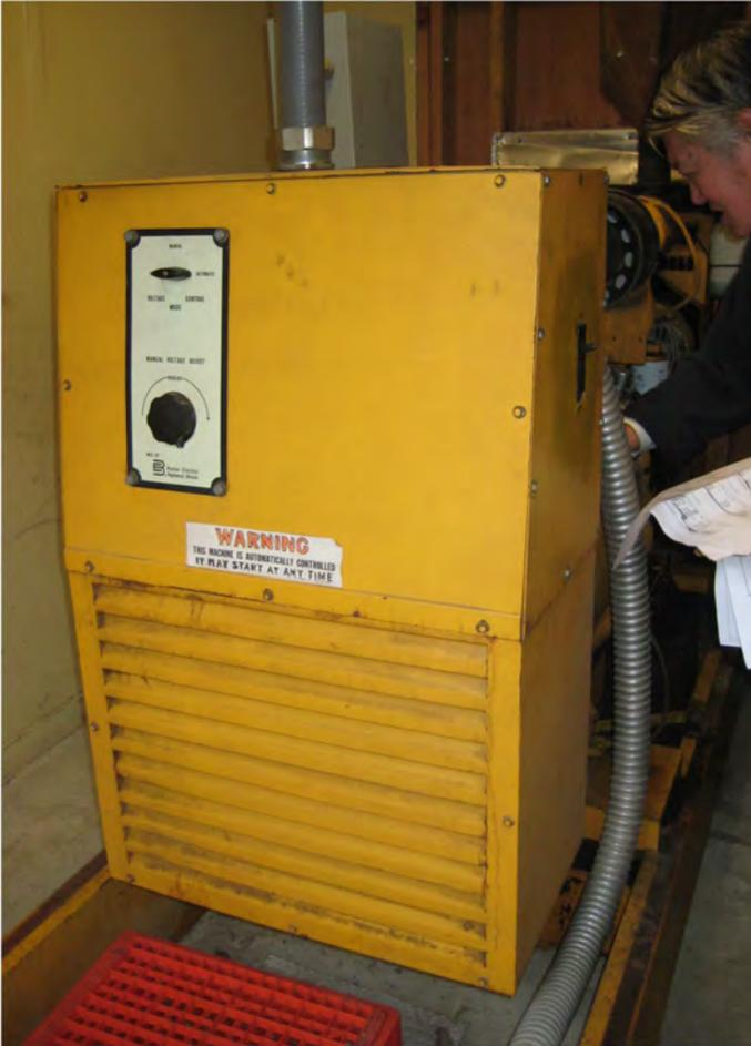
EE2 – Single phase diesel fuel standby generator
