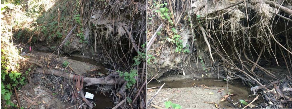
Figure 2 Undercutting near station 1+00
