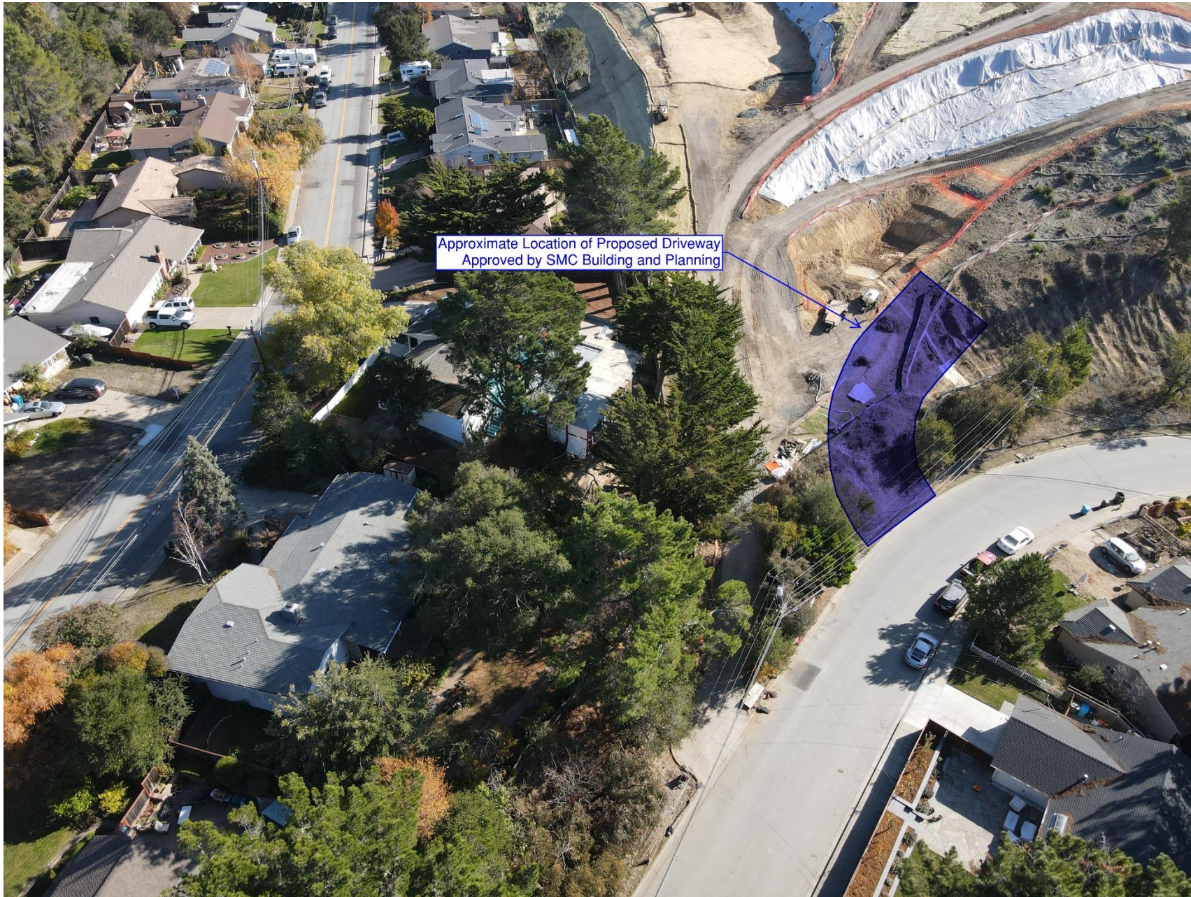
Figure 19: New driveway entrance
