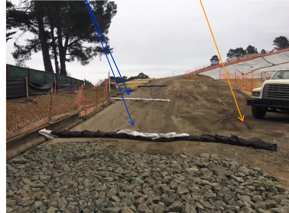
Figure 10: Installed Erosion Control Measures
