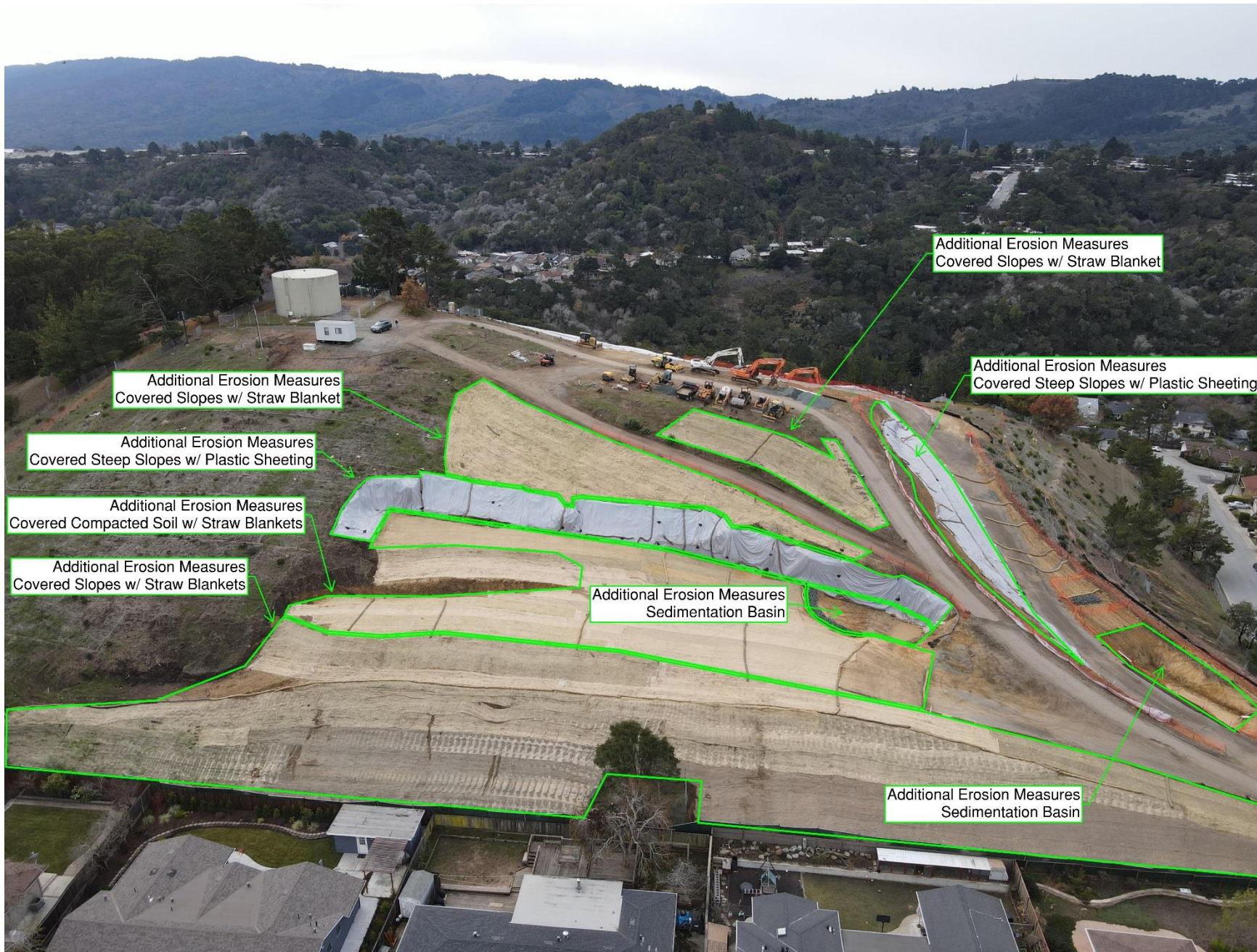
Figure 1: Construction Progress (North Side of Property)
