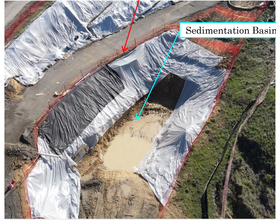
Figure 4: Installed Erosion Control Measures
