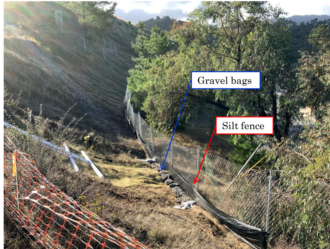
Figure 12: Installed Erosion Control Measures
