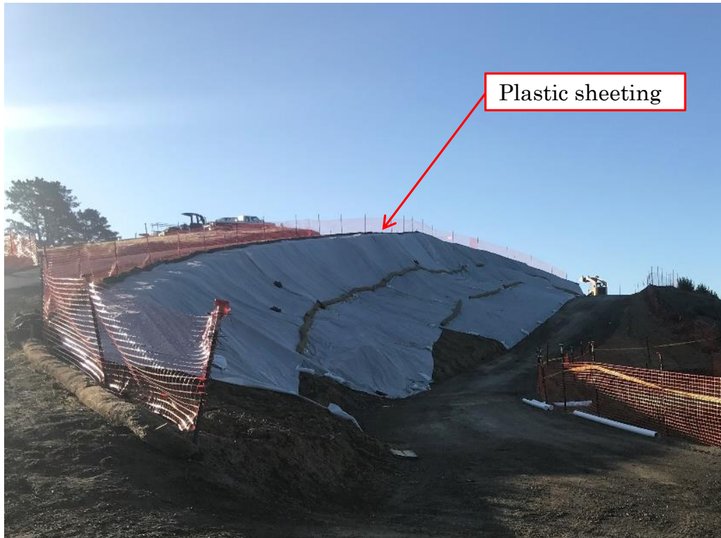
Figure 8: Installed Plastic Sheeting on Steep Slopes
