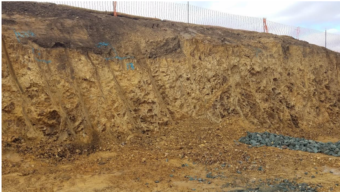
Figure 22: Excavated rock section (northern portion of site)
