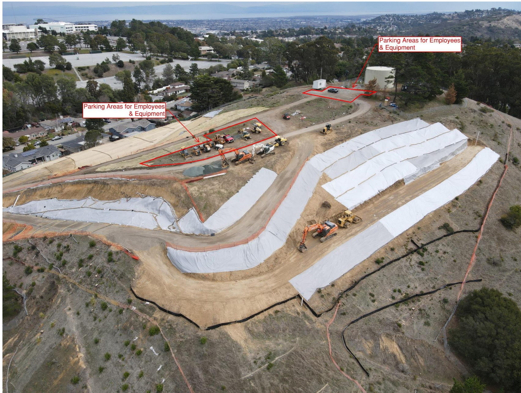
Figure 2: Construction Progress (South Side of Property)
