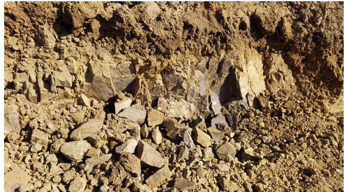
Figure 23: Excavated rock section (southern portion of site)
